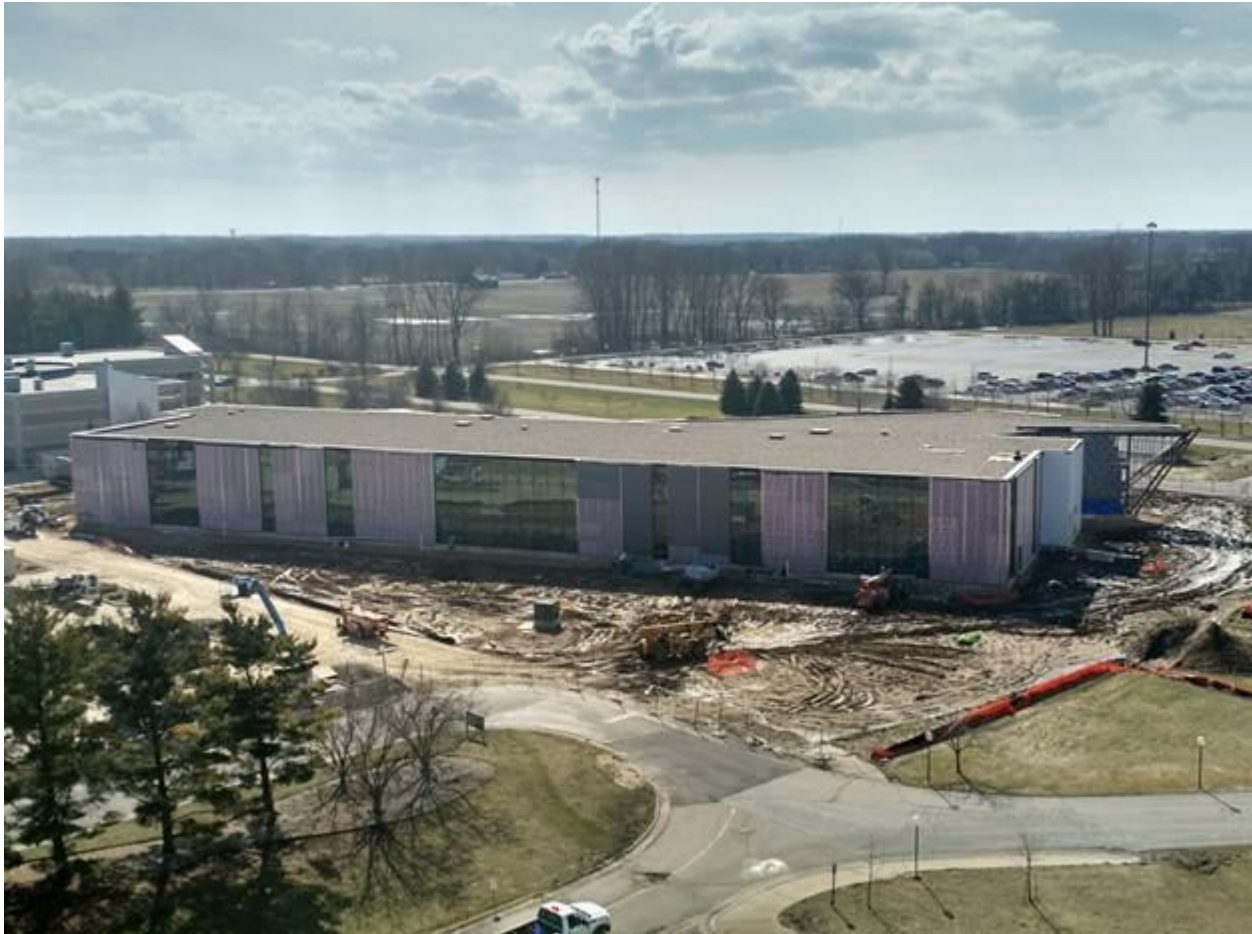
Hanson Technology Center: overhead view
