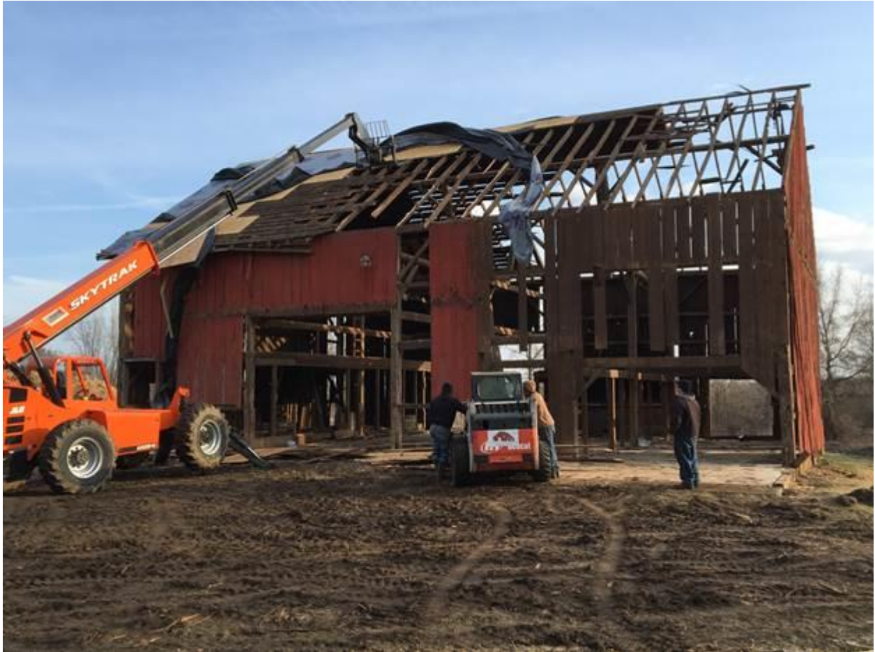
Barn Deconstruction: end of day 1
