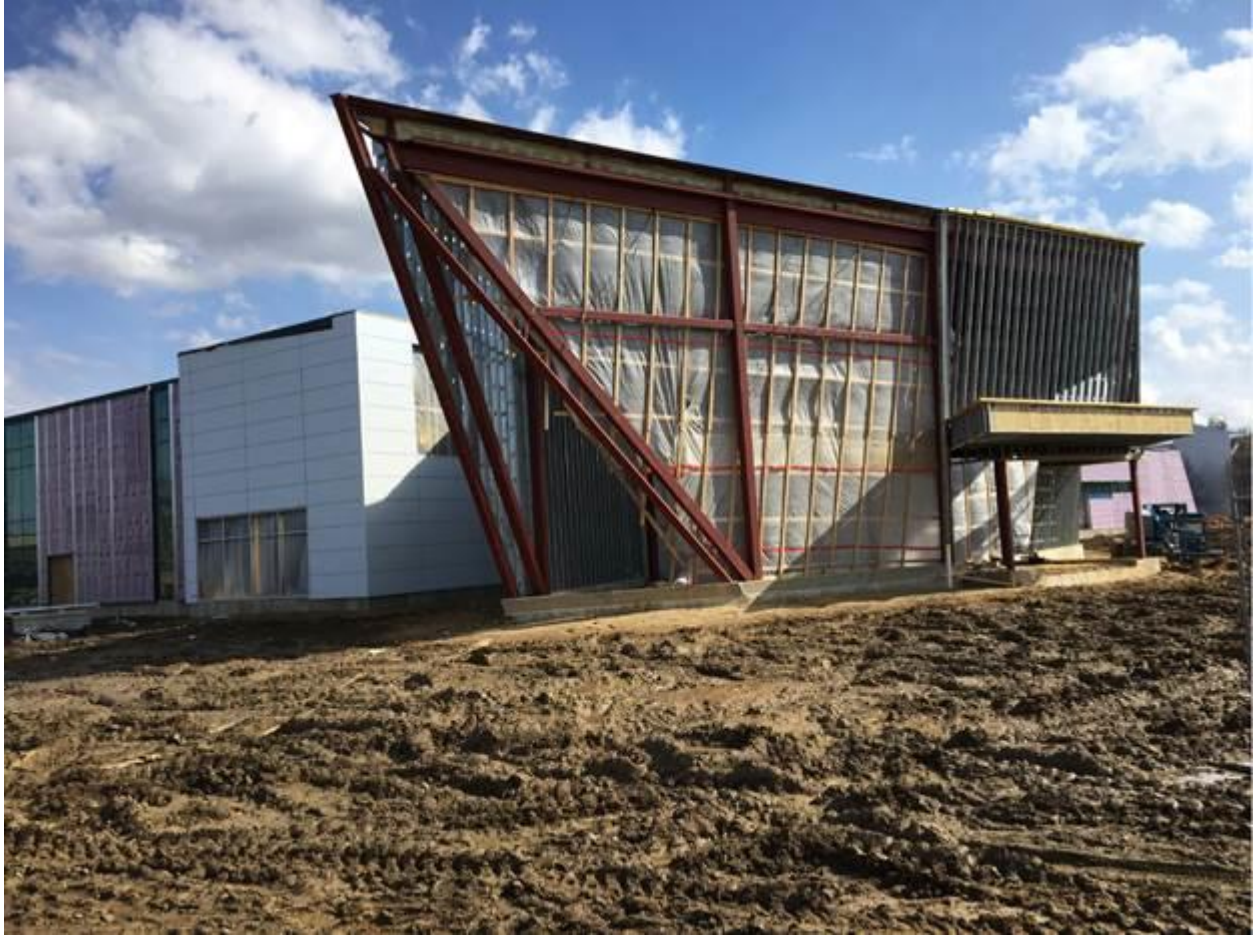
Hanson Technology Center: front entrance looking from Napier Academic front entrance
