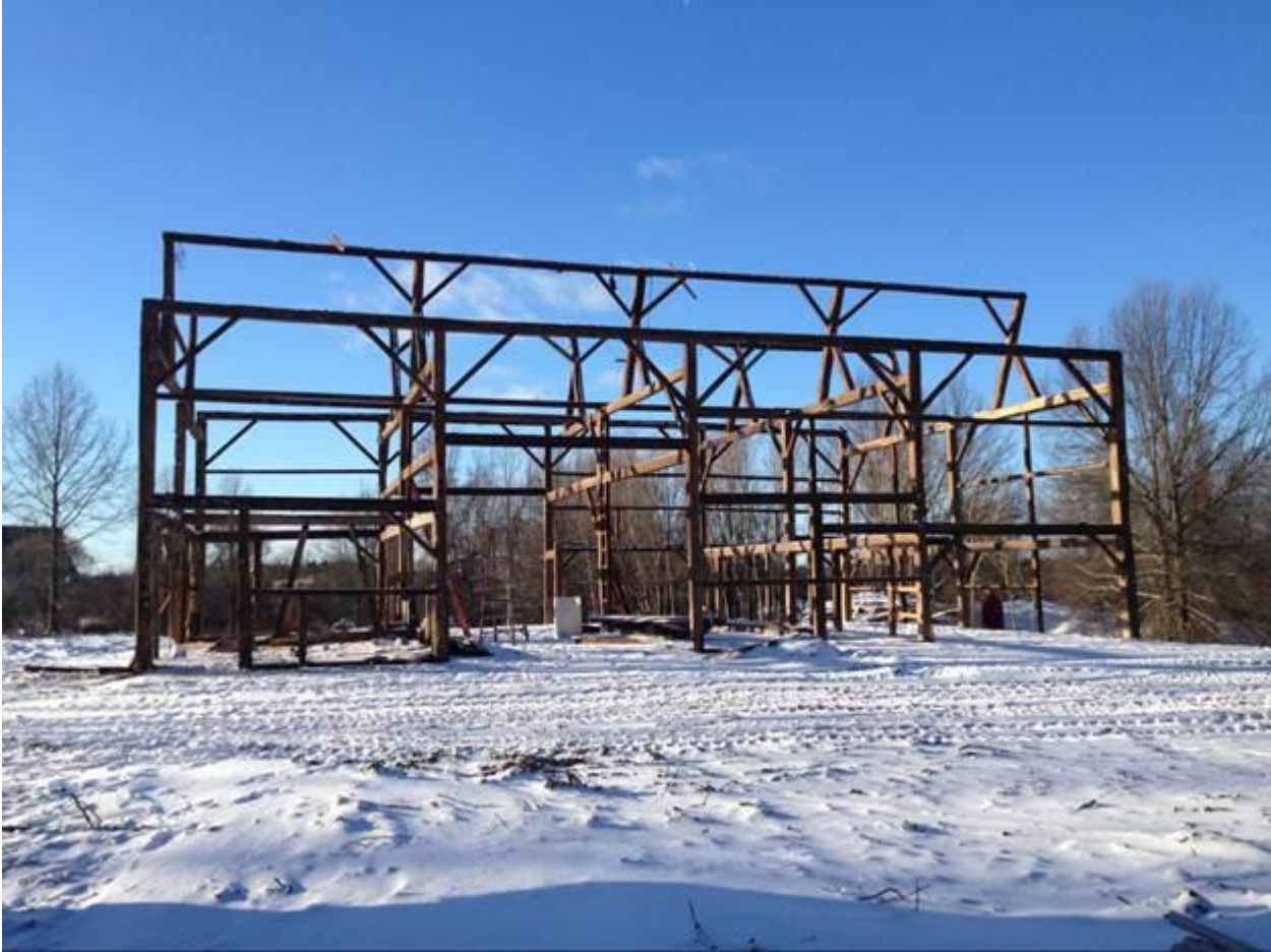
Barn Deconstruction: end of day 2. view from Empire Avenue
