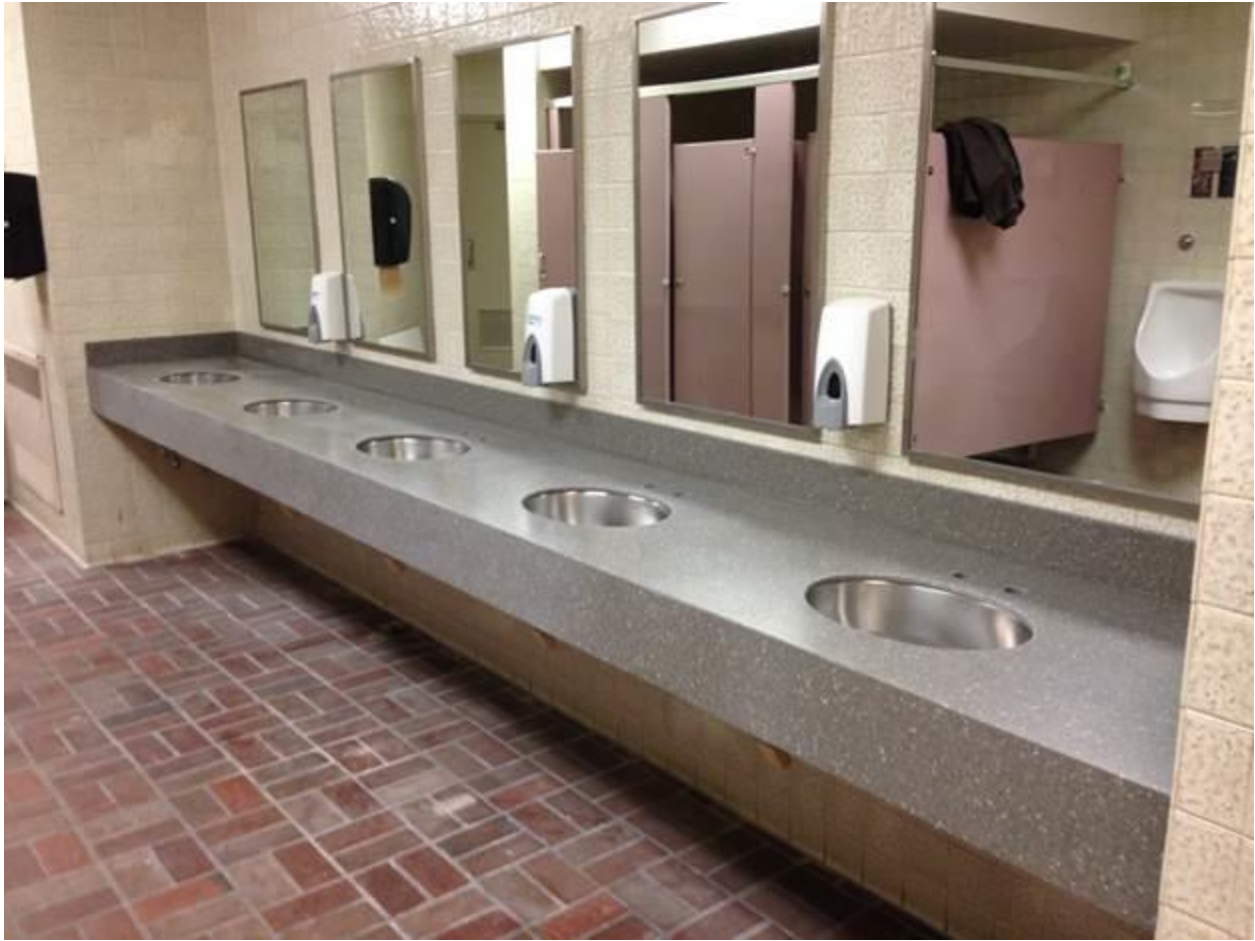
Upton Hall Restroom Renovation prior to completion
